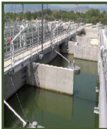
Basins at Boulder’s 75th St. Plant
