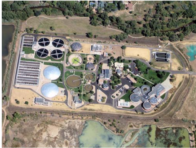
Boulder's 75th St. Wastewater Treatment Plant
